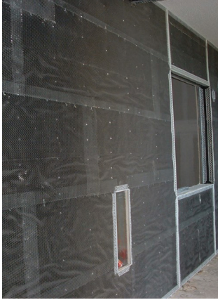
Metal lath attached to wall with PVC accessories.
